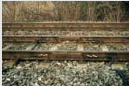
Connections of metallic structures to rails for grounding purpose
