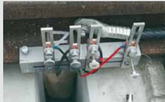
On site testing
